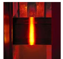
Rail weld after removal of the flash
